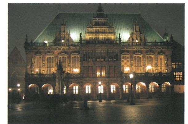
Town Hall with and without backlit windows (the latter was the intention of the masterplan)
